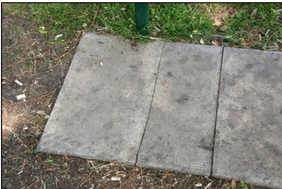
Fig. 5: Cracked slab in front of Bench S1.
