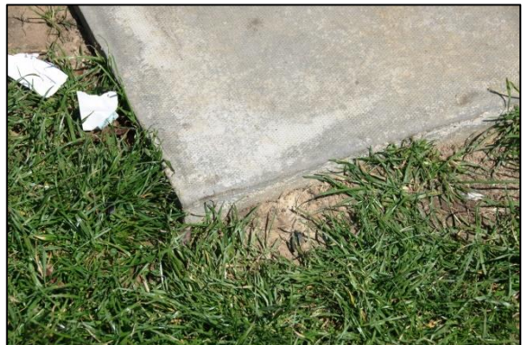
Fig. 6: Exposed corner of slab in Play Area.
