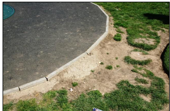
Fig. 12: Hazardous kerb on Roundabout.
