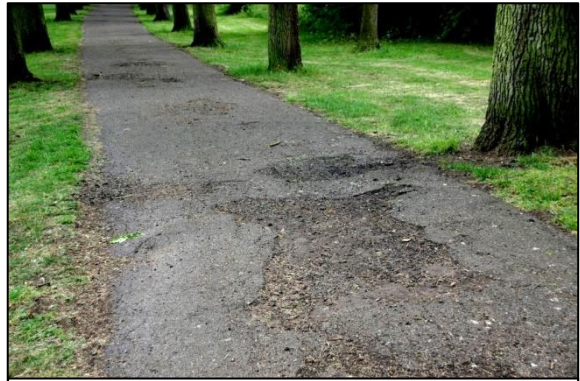
Fig. 2: Broken surface of Cedar Walk.
