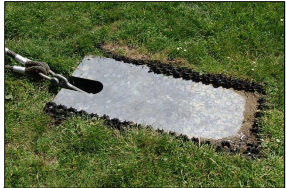
Fig. 10: Exposed anchor plate on Pyramid.
