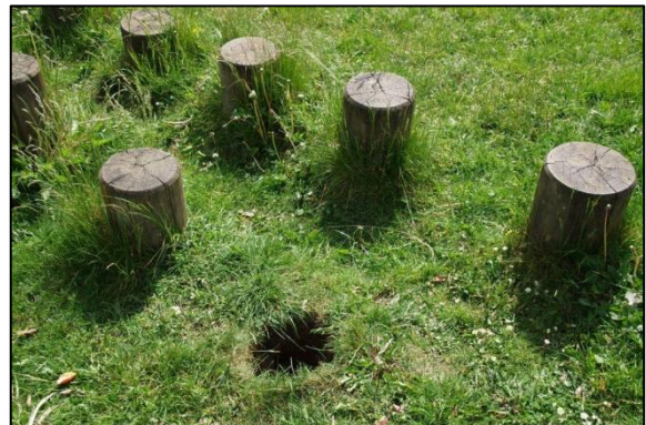
Fig. 14: Hazardous post hole on 'Monster'.
