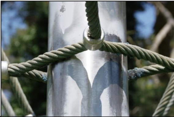
Fig. 9: Loose cables & pole on Pyramid.
