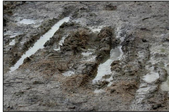
Figure 4: Mallard Walk (new 'all-weather' pathway) damaged by vehicles.
