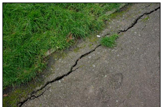
Figure 21: The tarmac on some older paths is showing signs of deterioration.
