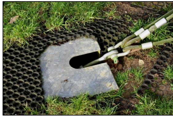
Figure 19: Exposed ground fixings for the climbing pyramid may represent a hazard.
