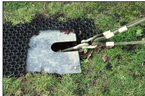
Figure 14: Exposed ground fixings for the climbing pyramid – January, 2017.
