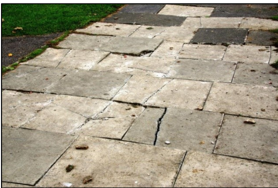
Figure 17: Damage caused to Greenside by Contractor's vehicles – October, 2016.
