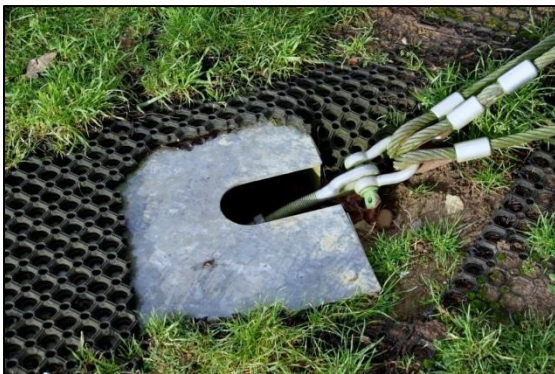
Figure 13: Exposed ground fixings for the climbing pyramid – January, 2016.
