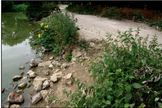
Fig. 18: Lake embankment in July showing severe erosion into Lake.
