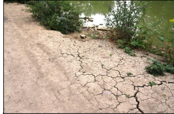
Fig. 19: Top of the Lake embankment in July showing cracks in surface.
